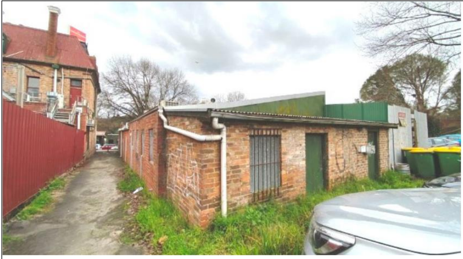
Figure 3 Site Rear Building facing North
